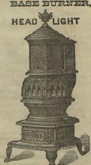
(AS WE GUARANTEE FOR IT) (Perfect Combustion of Fuel and Gases,) (Making little or no Soot or Cinder,) First-Rate Draft with entire control of the Fire,) GIVING A VERY STRONG AND UNIFORM HEAT.) nd the construction of the Stove is so simple that he parts which are exposed to intense heat can be easily and quickly replaced at a small cost by he most inexperienced person. We are there-ore confident that the HEADLIGHT is Unequalited in the special points of)
